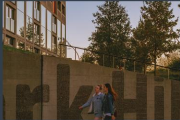
1 Transforming an architectural icon into a thriving, modern Community — Park Hill, Sheffield.
